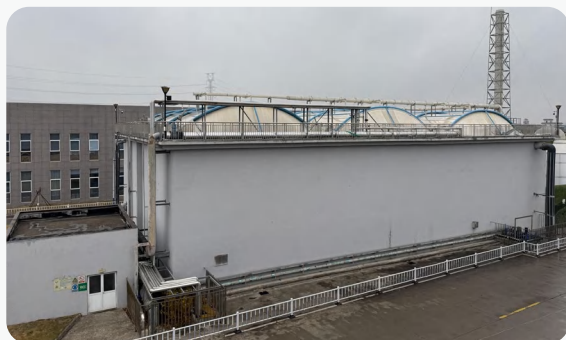
Wastewater Biochemical AO Treatment Tank
