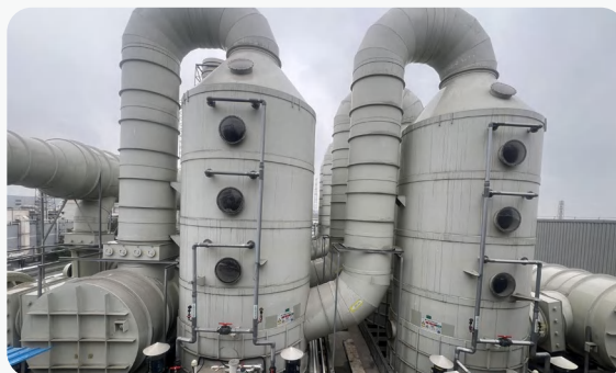
Waste Gas Treatment Unit: Acid Mist Tower
